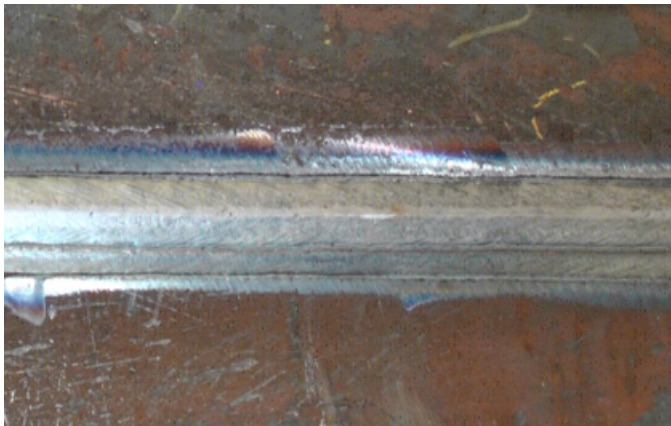
Fig. 1. A view of the face of weld made by 121 method in a PA position
