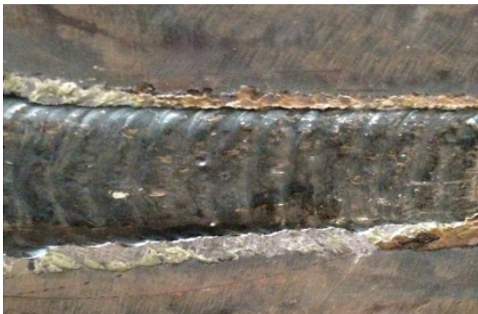
Fig. 2. A view of the face of weld made by 722 method in PF /g30 mm position
