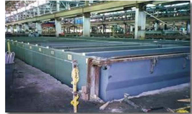
Copper Refining Cells
